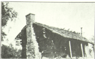
No. 1, shows one of the original buildings at Fort Coffee, built by the soldiers in 1834; it was afterwards used in connection with the Fort Coffee Academy.
