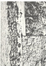
6. Portico wall at SW corner of building. Note portico pillars and of separate construction from portico wall.
