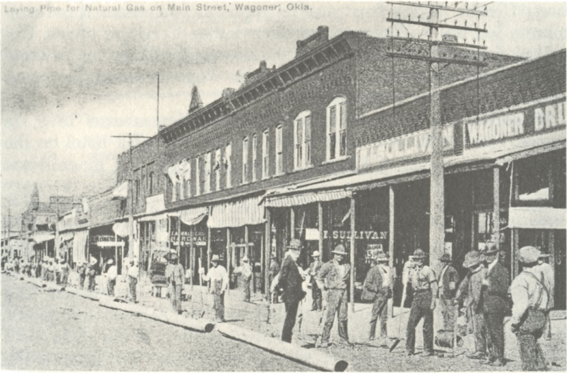
Laying Pipe for Natural Gas on Main Street, Wagoner, Okla.
