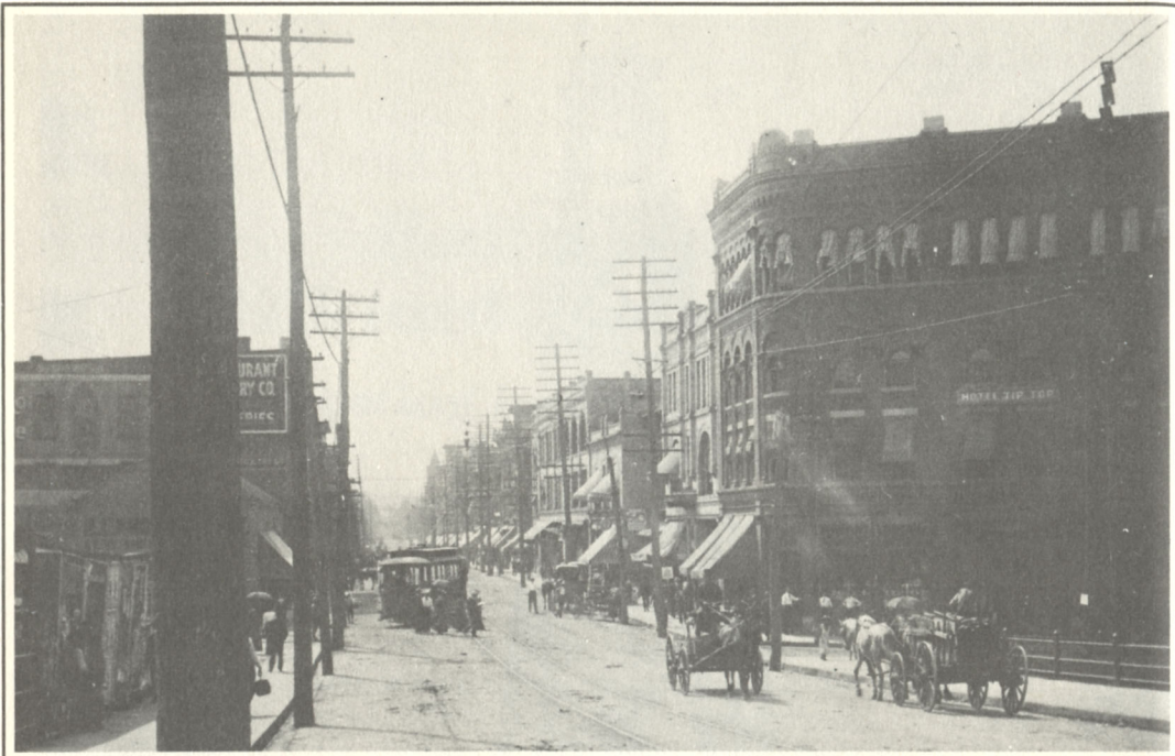
The Oklahoma Central Railway was conceived to bridge the open terrain between Durant (above) and Chickasha (below right). Agricultural prosperity and urban growth along the proposed line impressed Dutch investors (Courtesy Oklahoma Historical Society).
