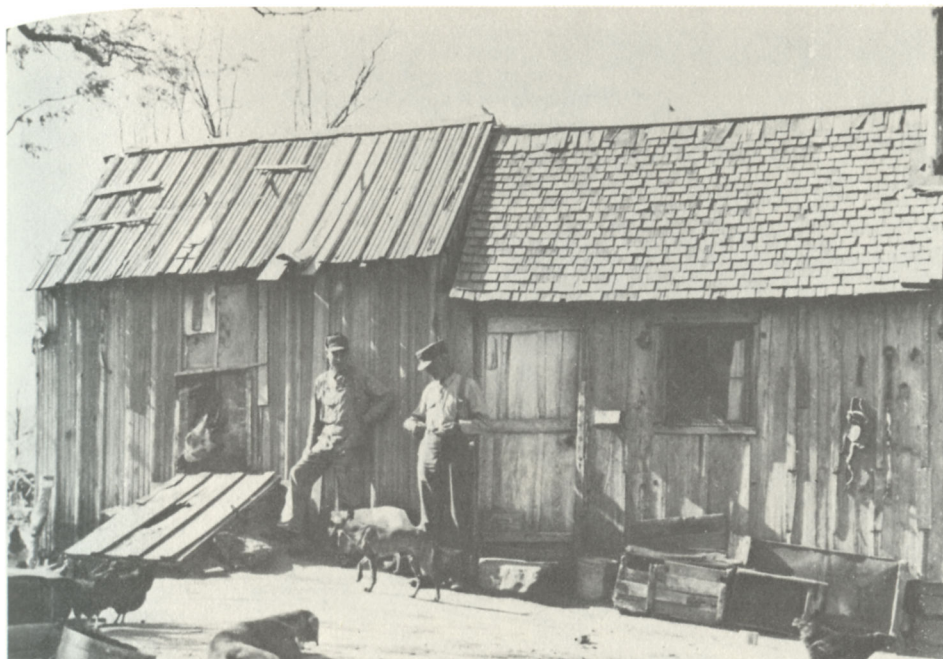
A farm near Reydon, Oklahoma. As late as the 1930s, many farms in Oklahoma still had no electricity, a problem the federal government tried to solve by creating power distribution systems (Courtesy Oklahoma Historical Society).
