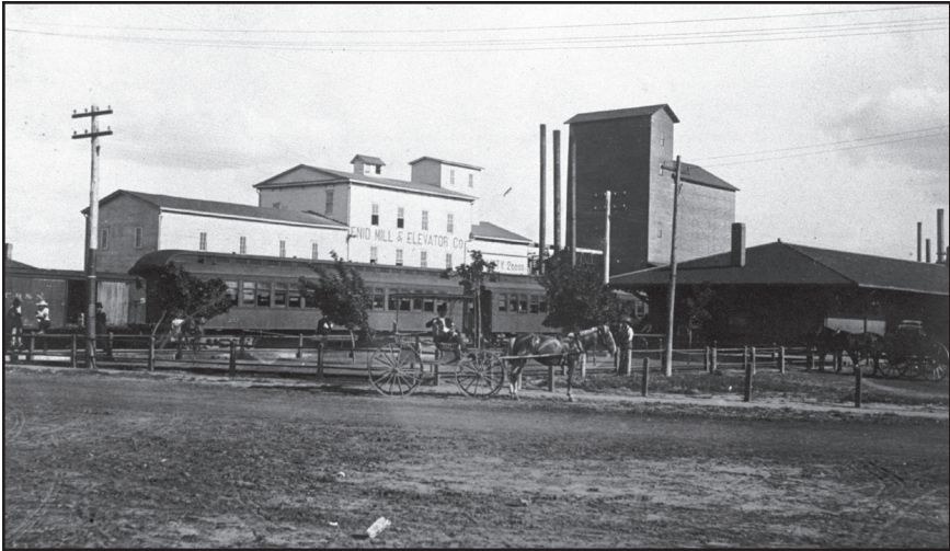
Enid railroad depot and Enid Mill and Elevator Company (19413.90.31.14, Cherokee Strip Museum Collection, OHS).
