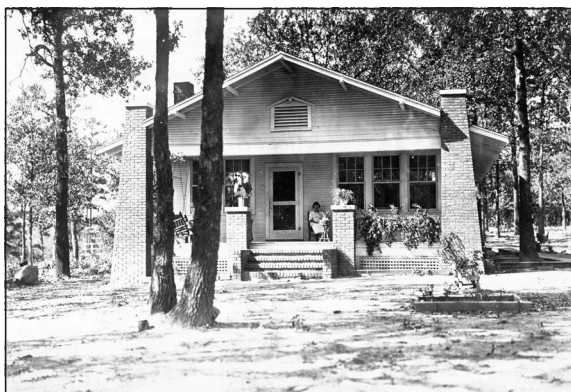
Superintendent's house at the Eastern Oklahoma Tuberculosis Sanatorium near Talihina (photograph courtesy of the author).
