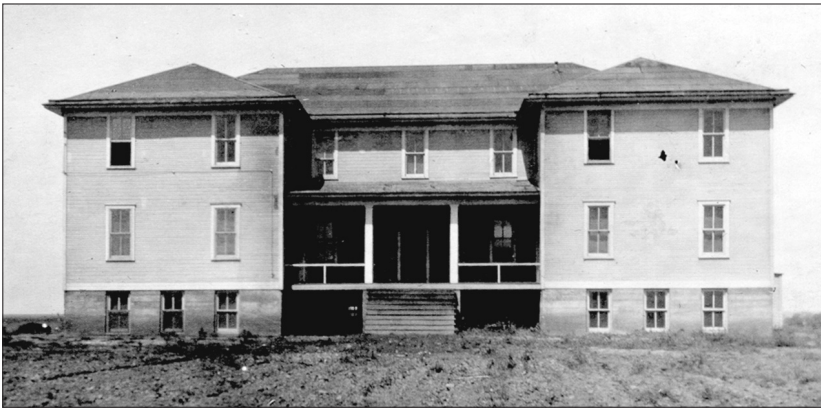
Cameron's women's dorm, newly constructed (OHS Research Division photo).
